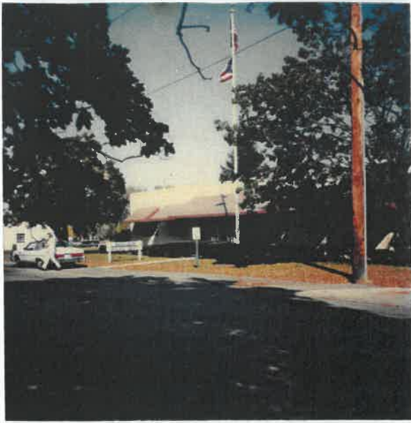
Police Station Replastering and painting
